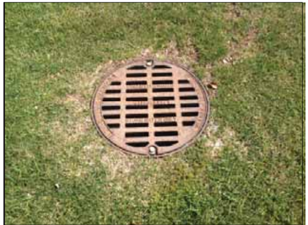
Drywell Cleaning - multiple retention areas 27 total
