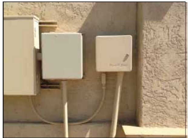
Rainbird Irrigation Station - multiple locations 26 total
