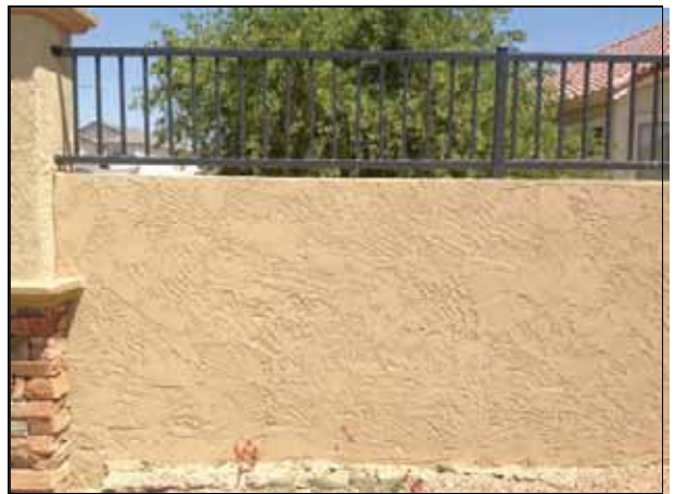
Perimeter Wall and Wrought Iron painting
