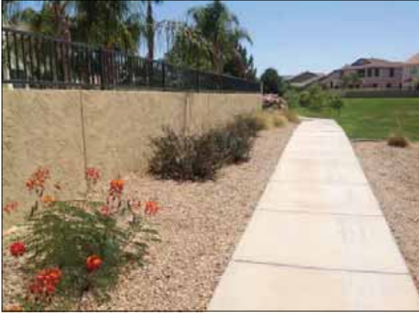
Perimeter Wall and Wrought Iron painting
