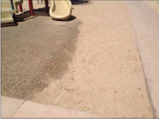
Tot Lot Nicolet - playstructure, sand, totlot surface, trash, trellis and picnic tables
