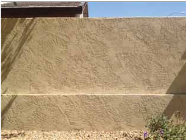
Perimeter Wall and Wrought Iron painting
