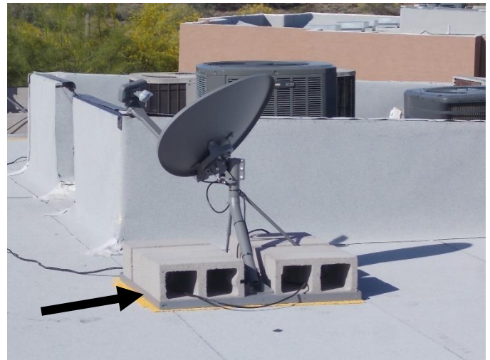
Protective slip sheets should always be installed between the roof system and any type of equipment platform or support.
